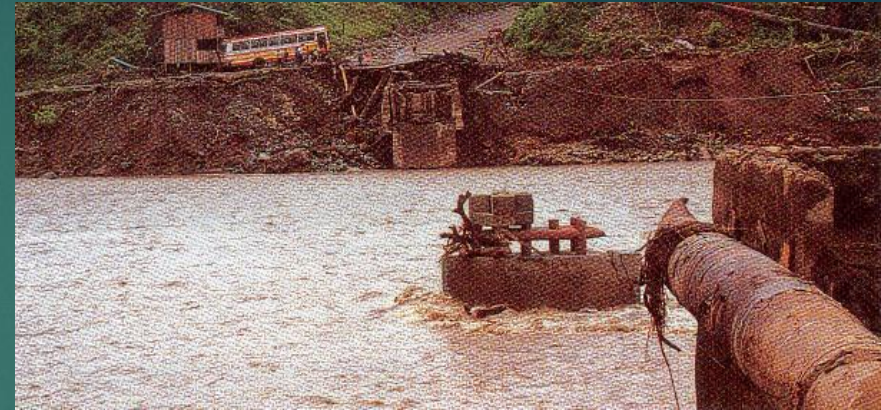
Damage to the oil pipe
