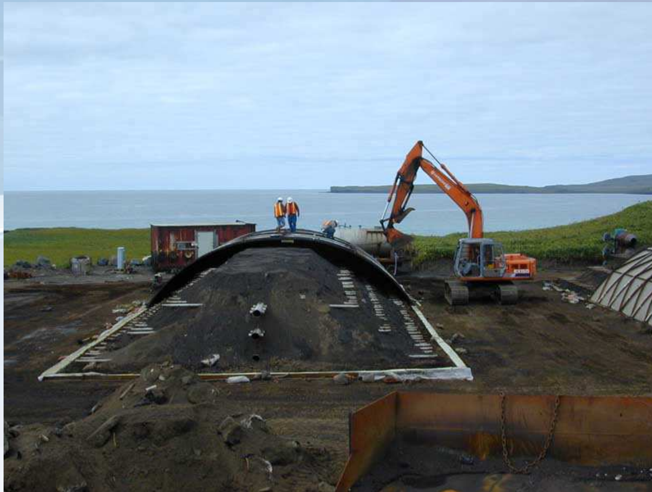
Soil remediation by thermal conduction, St. Paul Island
