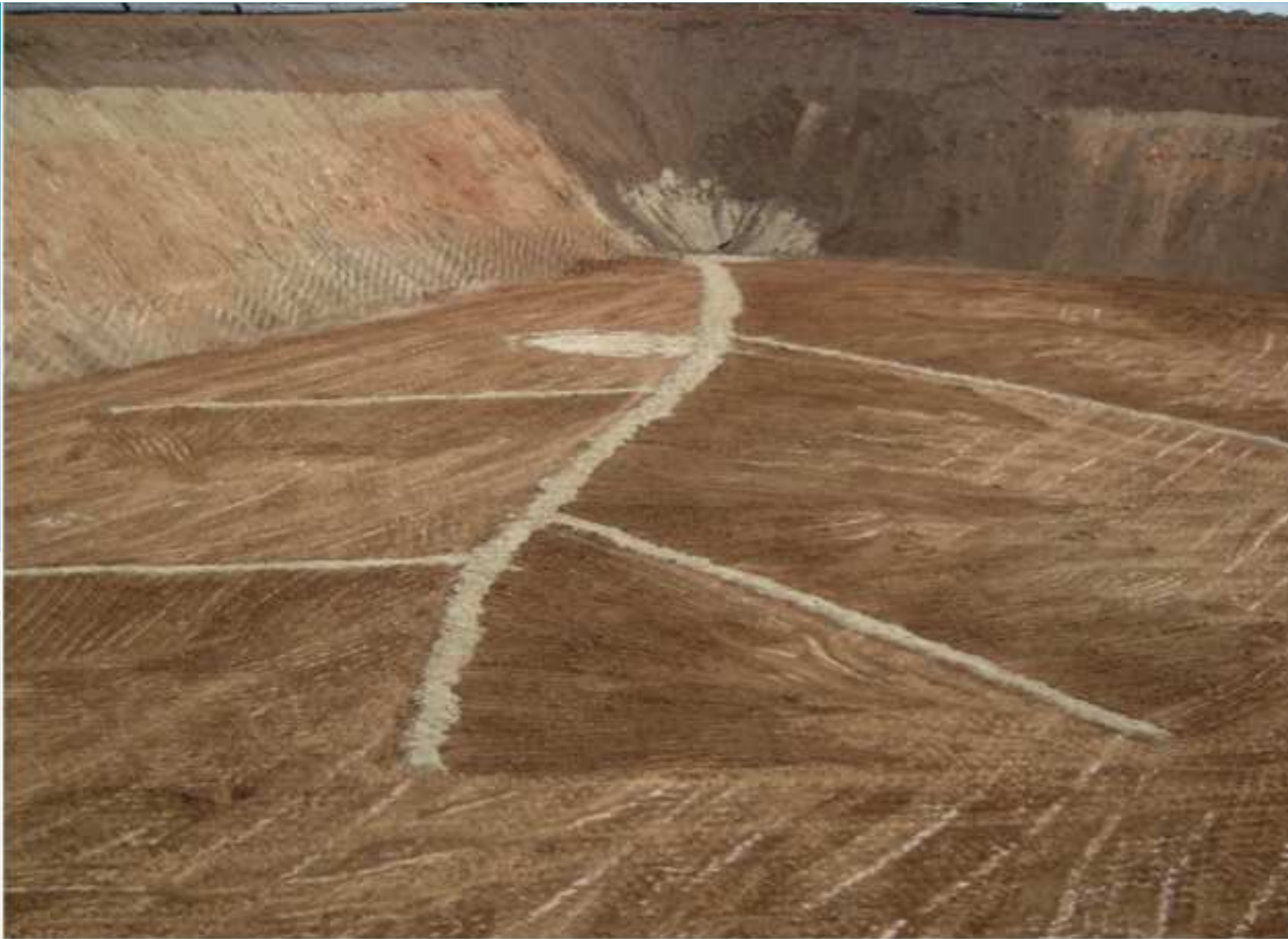
Drainage installation
