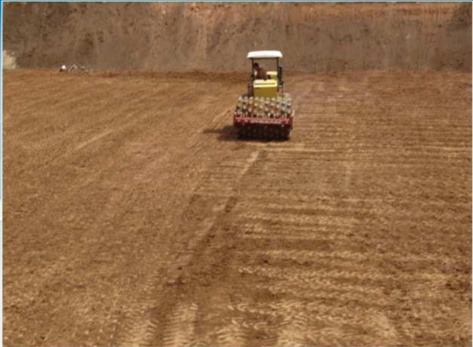
Soil compaction
