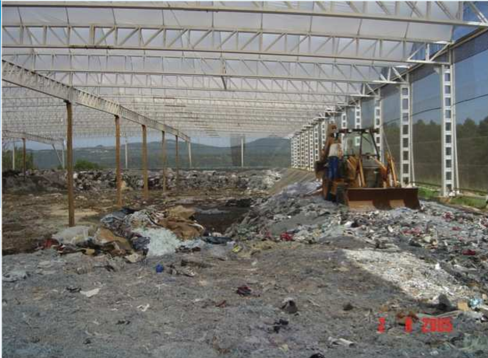
Pit in operation
