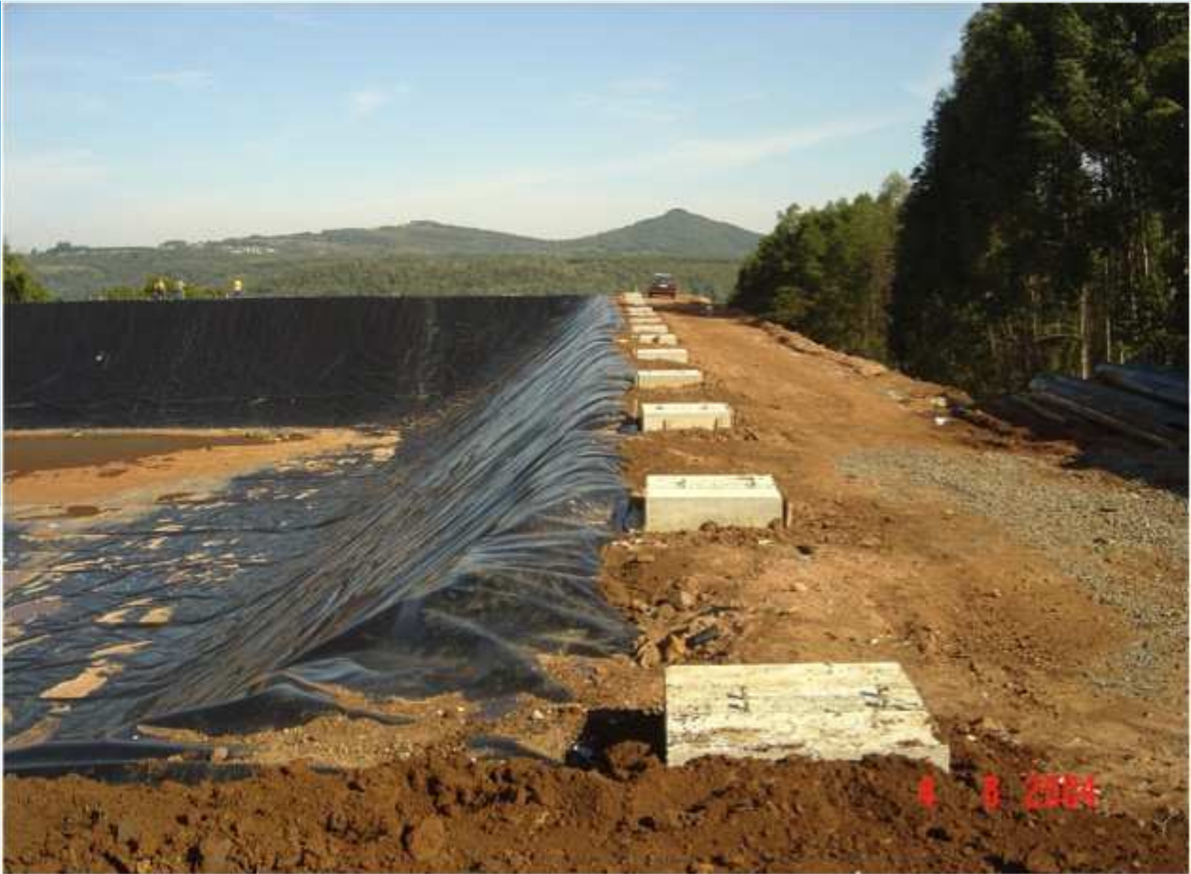
Foundations for cover
