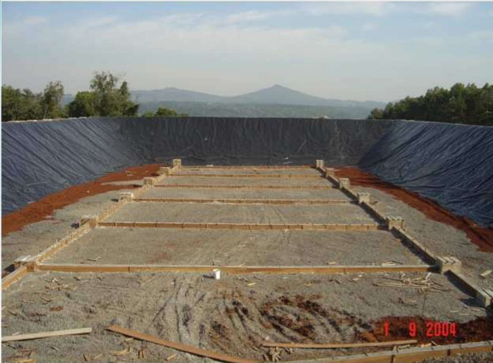
Base of the roof metal structure
